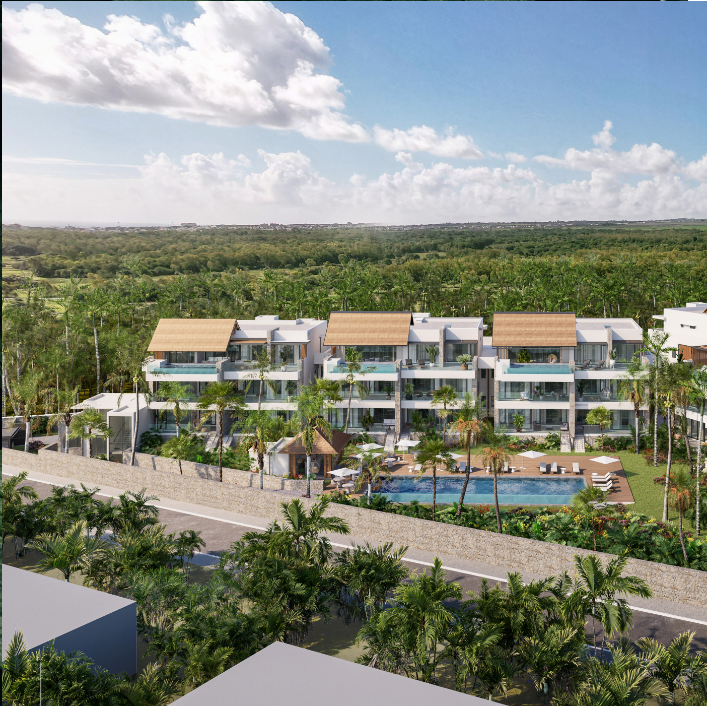
Aerial view of the project
